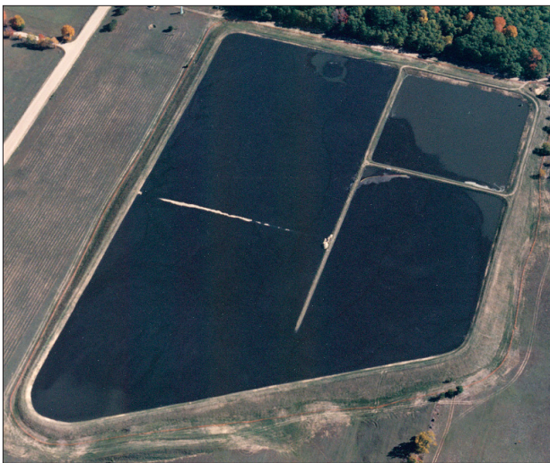
Figure 11. Dredge material disposal cell.
