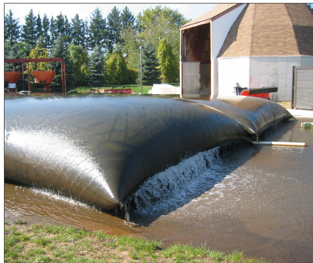
Figure 12. Geotextile tubes for disposal of dredged material.
