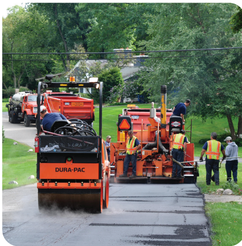
Township road crews working to resurface a residential road in the Township.
